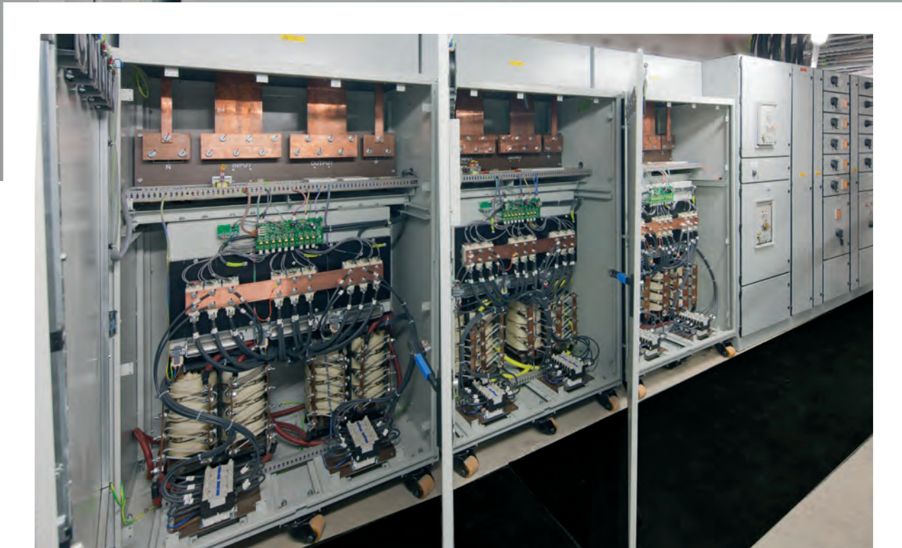
Seamless bypass arrangement. Fully integrated low voltage panel with three phase 2,400Amps / 1,584kVA
